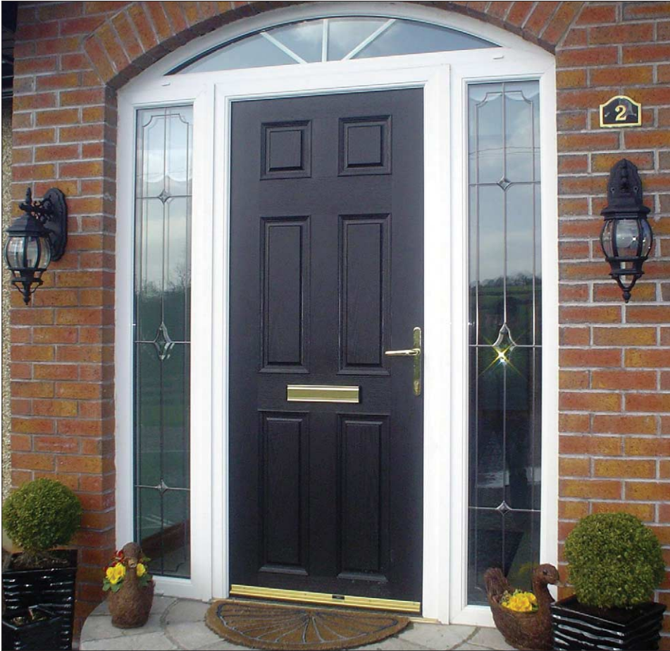
Typical door set manufactured by New World Developments. The adoption of Scott Bader Crystic Crestapol 1210 resin has enabled door skin mouldings to be produced quicker, to higher standards of finish and with lower rejection rates.
